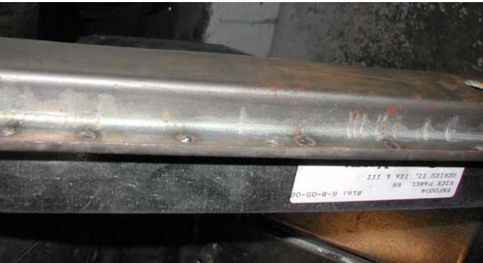
(Figures 8 & 9) Here you can see that the reproduction doorposts are constructed differently than the originals. The replacement (top) has a separate outer face that is spot welded to the vertical sections. The original (bottom) is formed from one piece of steel. The bottom of the post (not the foot) is also simplified on the repair section and differs from the original in detail. The profile of the post is close enough that a clean repair can be achieved without making your own section. (photos taken from the completed firewall)
