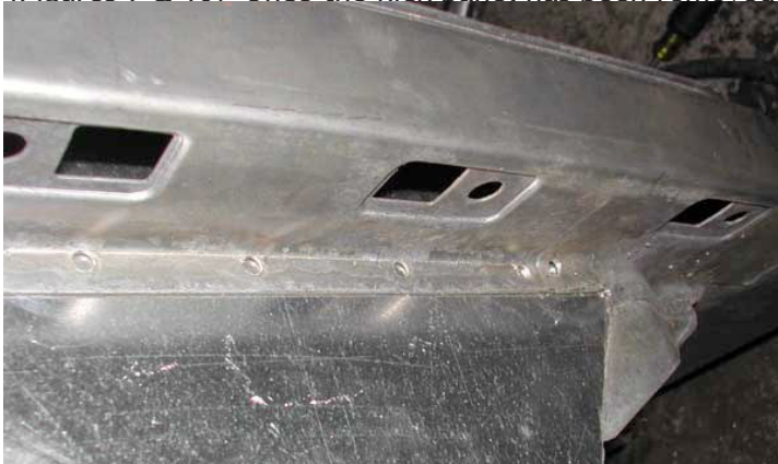
(Figures 9 & 10) Once the kick panel has been removed
