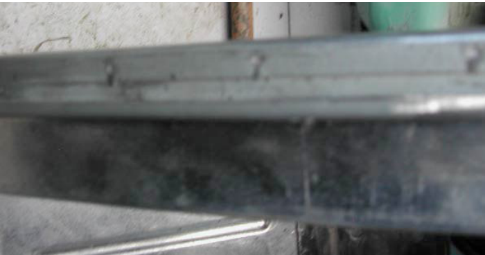
(Figure 7) Replacing the door post and ensuring an accurate fit is important. An angle iron jig should be used to ensure the correct spacing of the doorposts. A simple jig consisting of section of angle with holes in both ends which the door posts can bolt to is sufficient to ensure correct spacing.
