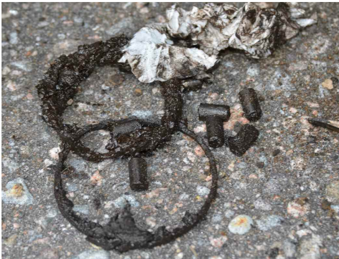
The broken bearing in Quebec
