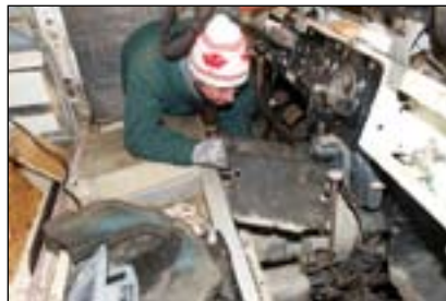
Finally, Installing the floors
