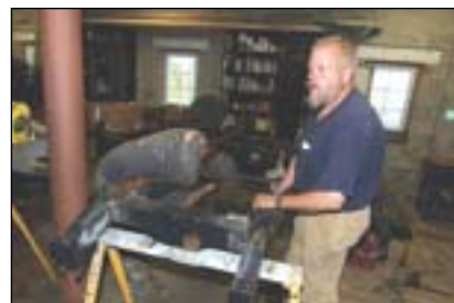
Bill O'Hara assisting Dave Bobeck moving the centre cross member back into place. It was moved back six inches and down three to make room for a V6 conversion.
