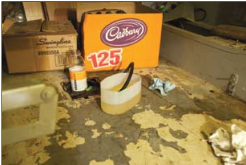
Temporary fuel supply
