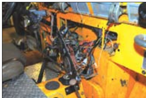
The rest of the wiring harness was not much better!
