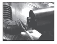
air intake on top and not underneath as designed. This requires me to grind out the steel straps that hold the can in place so they'll fit around the fresh air intake opening ... as you
