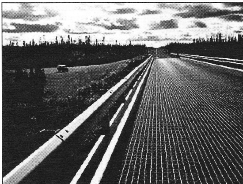
Bridge crossing the (diverted) Churchill River (near Churchill Falls). (Robert St-Louis)
